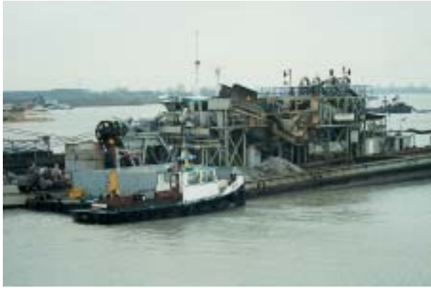
HAVER-CPA Online application on a dredge
